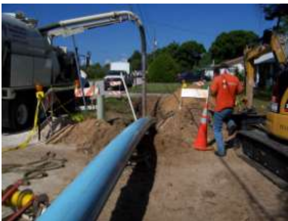
Photo from Clay Blvd. water main replacement project.
